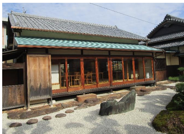
Photo 3: The Yokoyama Family Residence study and connecting corridor.
